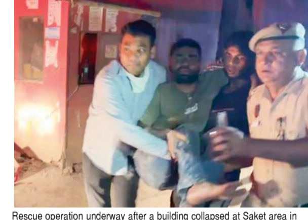
Rescue operation underway after a building collapsed at Saket area in New Delhi on Saturday
